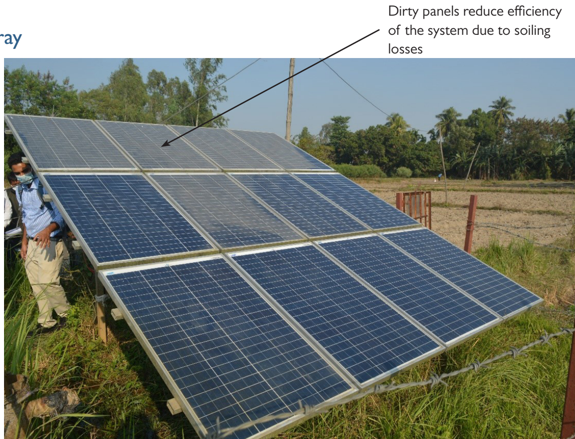
Figure 27 PV Array Maintenance (ecoPlanetenergy, 2016)
